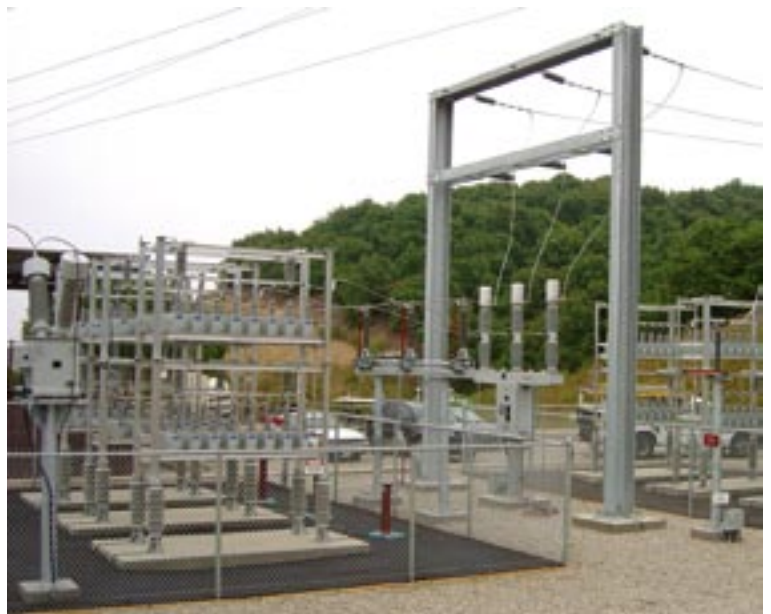
CapSwitcher® 72.5 kV installed on a capacitor bank
