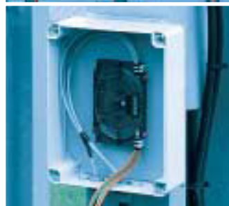
Temperature measurement. Sealing end box for temperature measurement by means of optical fibres in the cable sheath.
