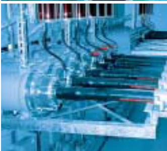
TF 1.170-11 Sealing end for single-pole insertion in SF6 switchgear.
