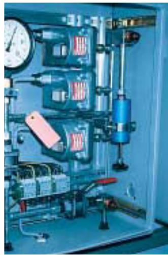
All under control. Pressure control box for oil-filled cables with pressure gauge, pressure switches and pressure pump.
