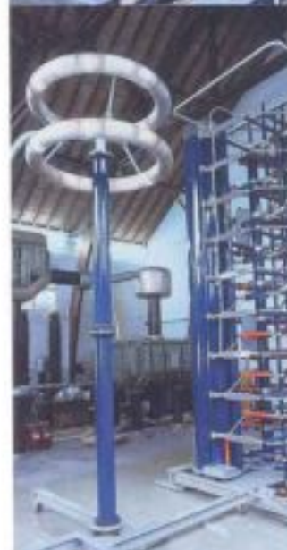
Test passed. Our test field for type testing according to IEC.
