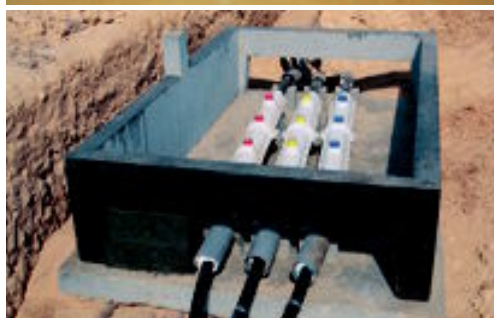
Laying in a pit. Joints with protection box in a concrete pit.
